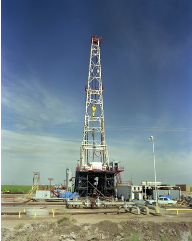
Photo by Warren Gretz, NREL/PIX 00450
