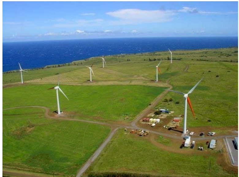
Figure 4. Hawaii Renewable Development, owned by HRD LLC and located at Upolu Point near the northern tip of the Big Island. The project utilizes 16 Vestas V-47 660-kW turbines spread over approximately 250 acres.
