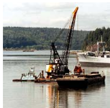
Dredging the confined aquatic disposal pit
