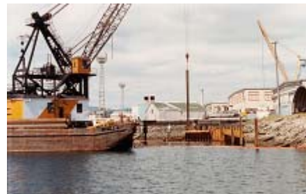
Installing sheetpile wall at Site 1
