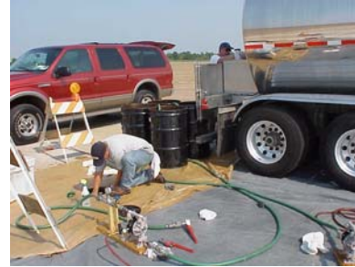
Personnel monitor the injection process
