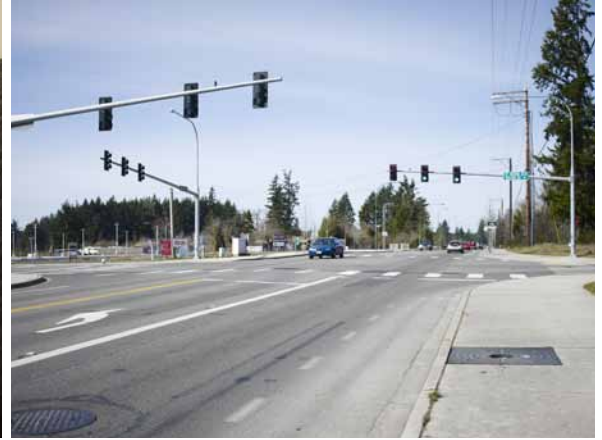
Killion Road LID Financing Thurston First Bank, Yelm, Washington
