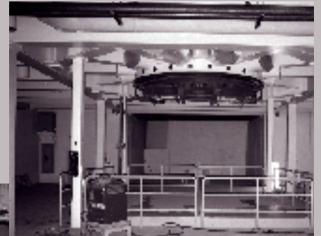
PBFA II, basement looking at stack, 1984.
