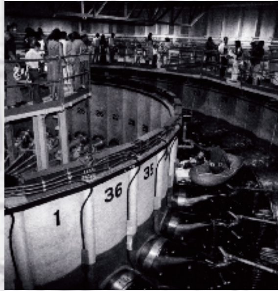
The crowd assembled for the 1980 dedication of Sandia's Particle Beam Fusion Accelerator (PBFA I) watches technicians at work in the water around the machine. It accelerated light-ion beams for Sandia's inertial confinement fusion experiments aimed at producing abundant, economical energy during the 21st century.
