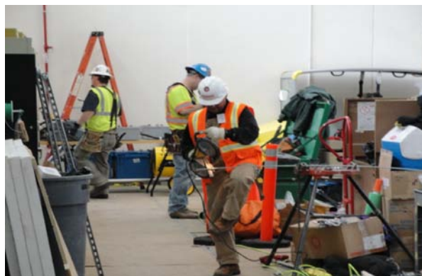
Workers installing chilled water and electrical components in TTF laboratory
