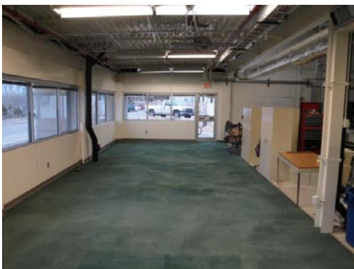
TTF laboratory before construction
