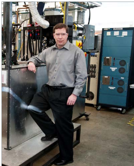
Senior Engineer Matthew Keyser with the Large Volume Battery Calorimeter connected to a battery tester in the back. Photo by Dennis Schroeder, NREL
