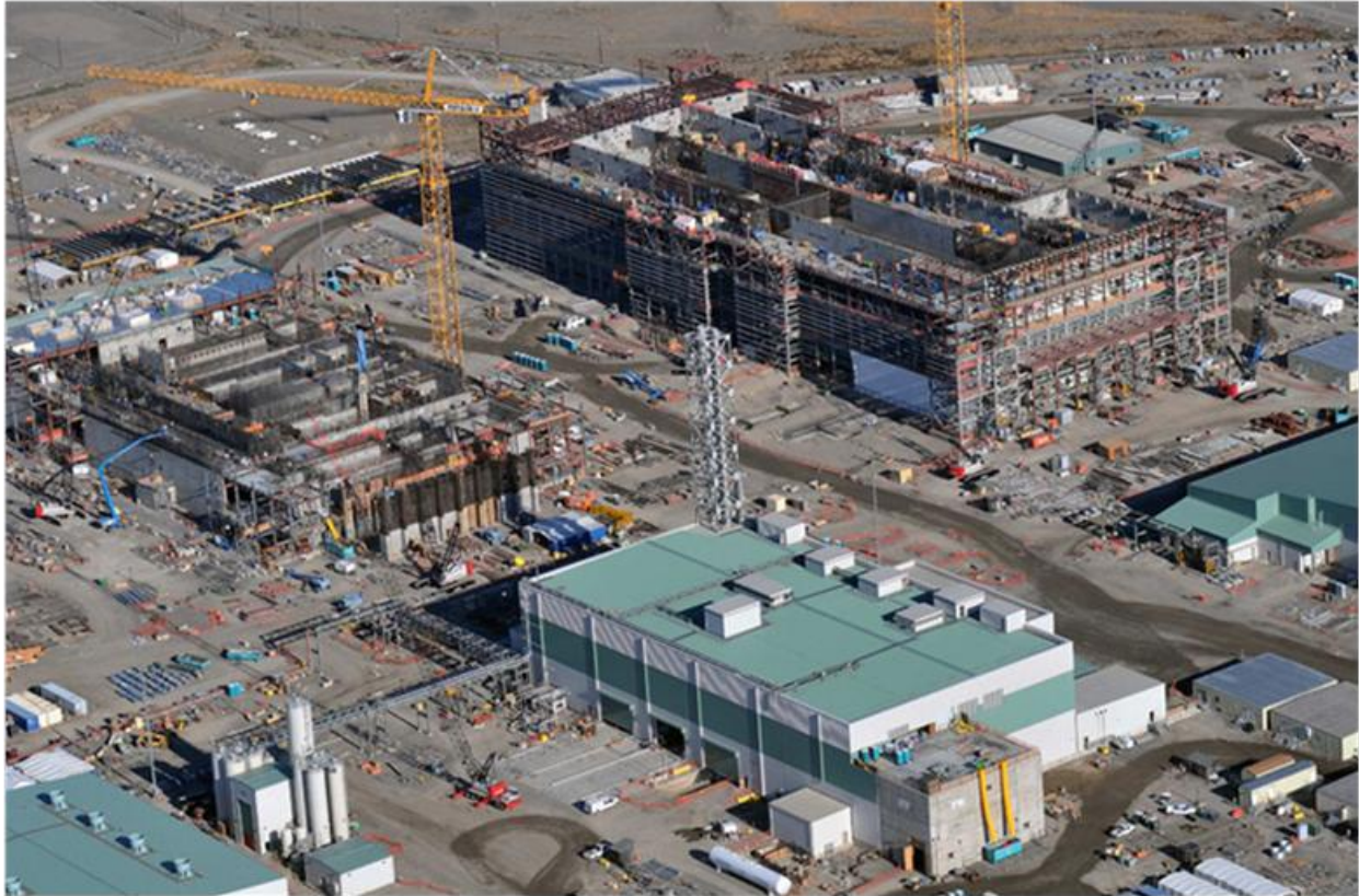
Figure 5-2. Aerial Photo of Waste Treatment and Immobilization Plant from the Southeast (August 2011)
