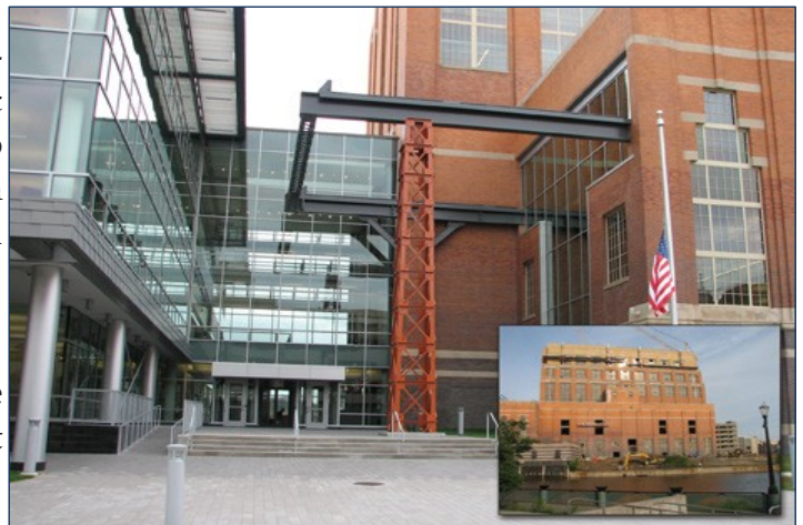
An economic development advance was used to renovate a 1938-era vacant power plant to create the new headquarters of Accident Fund Insurance Company in downtown Lansing, Michigan. The project will create 250 jobs and retain 622 jobs (before and after photographs).
