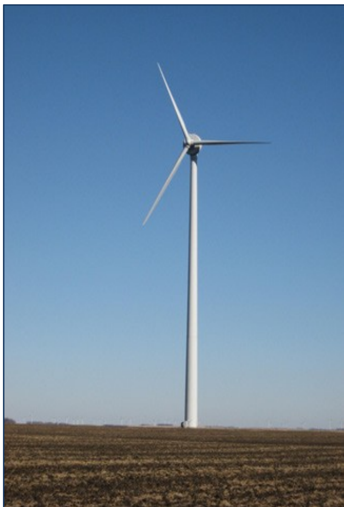
A community investment advance funded the construction of Woodstock Municipal wind system in Woodstock, Minnesota. The turbine has been linked directly to an electrical feeder supply line that provides the community with renewable energy.
