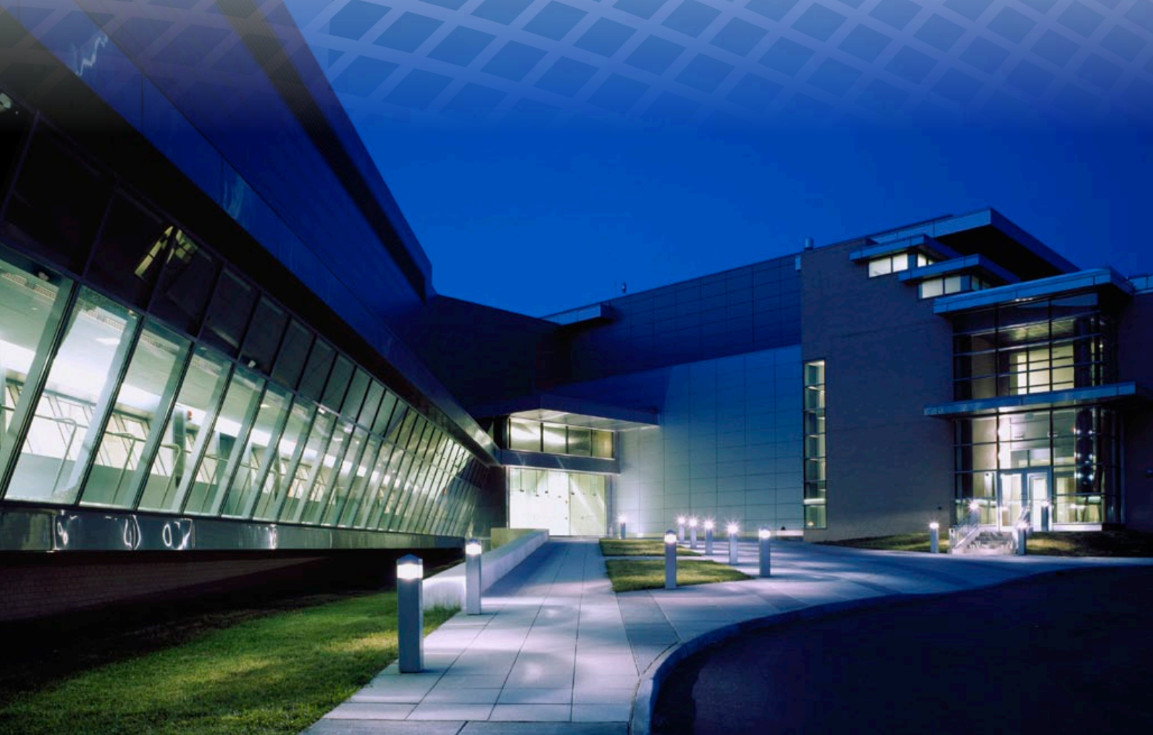
(Credit HDR Architecture, Inc./Steve Hall © Hedrich Blessing)
