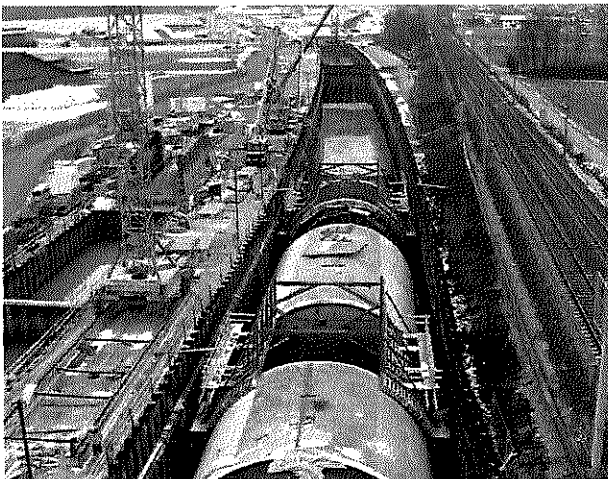
Photo: Job site at the lower Inn valley railway Radfeld centre
