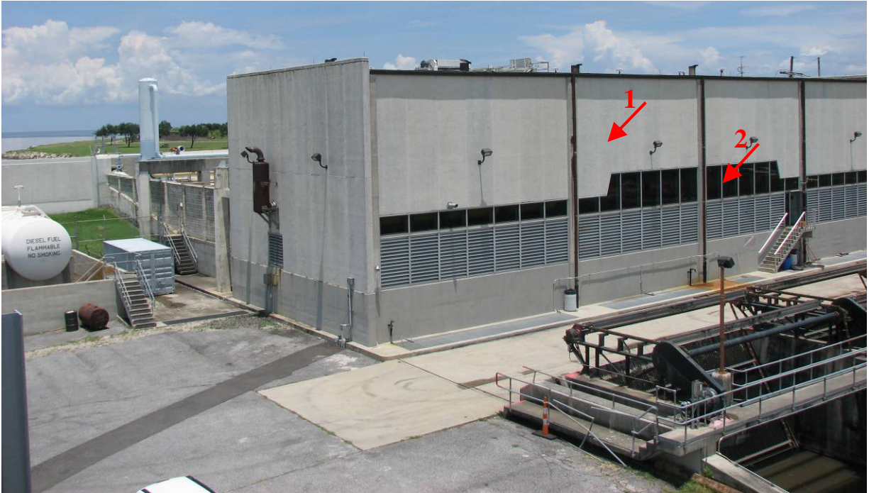
Figure 5: Bonnabel pump station is proposed for stormproofing to resist storm force winds. Features include: (1) precast concrete walls (2) windows
