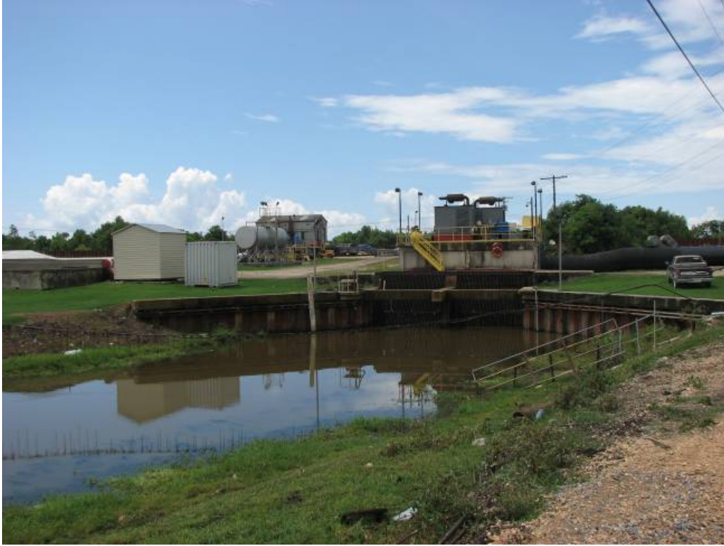
Figure 10: Lake Cataouatche pump station and surrounding habitat.
