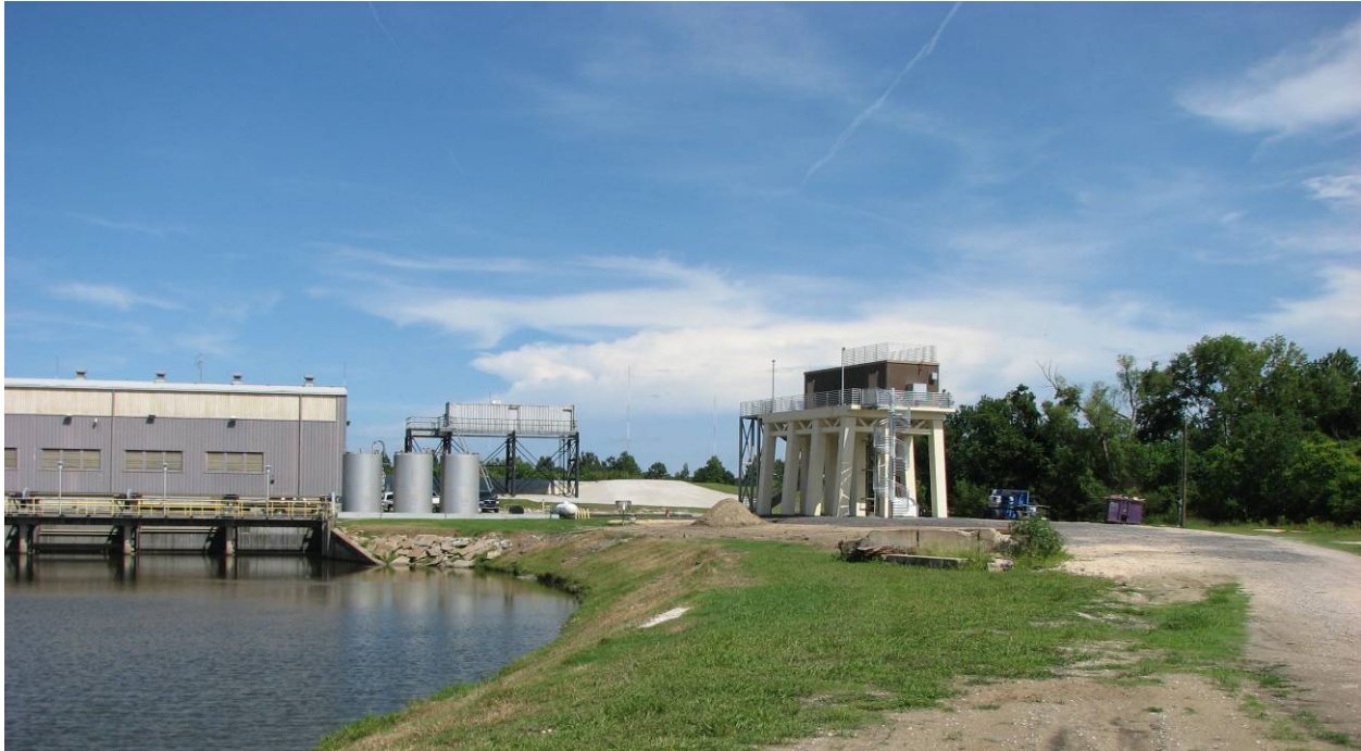
Planters Pump Station in Jefferson Parish, Louisiana (photograph taken on July 9, 2008).
