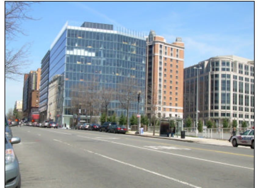
Photo Seventeen: View north to New York Avenue from 11 th Street and H Street, NW.
