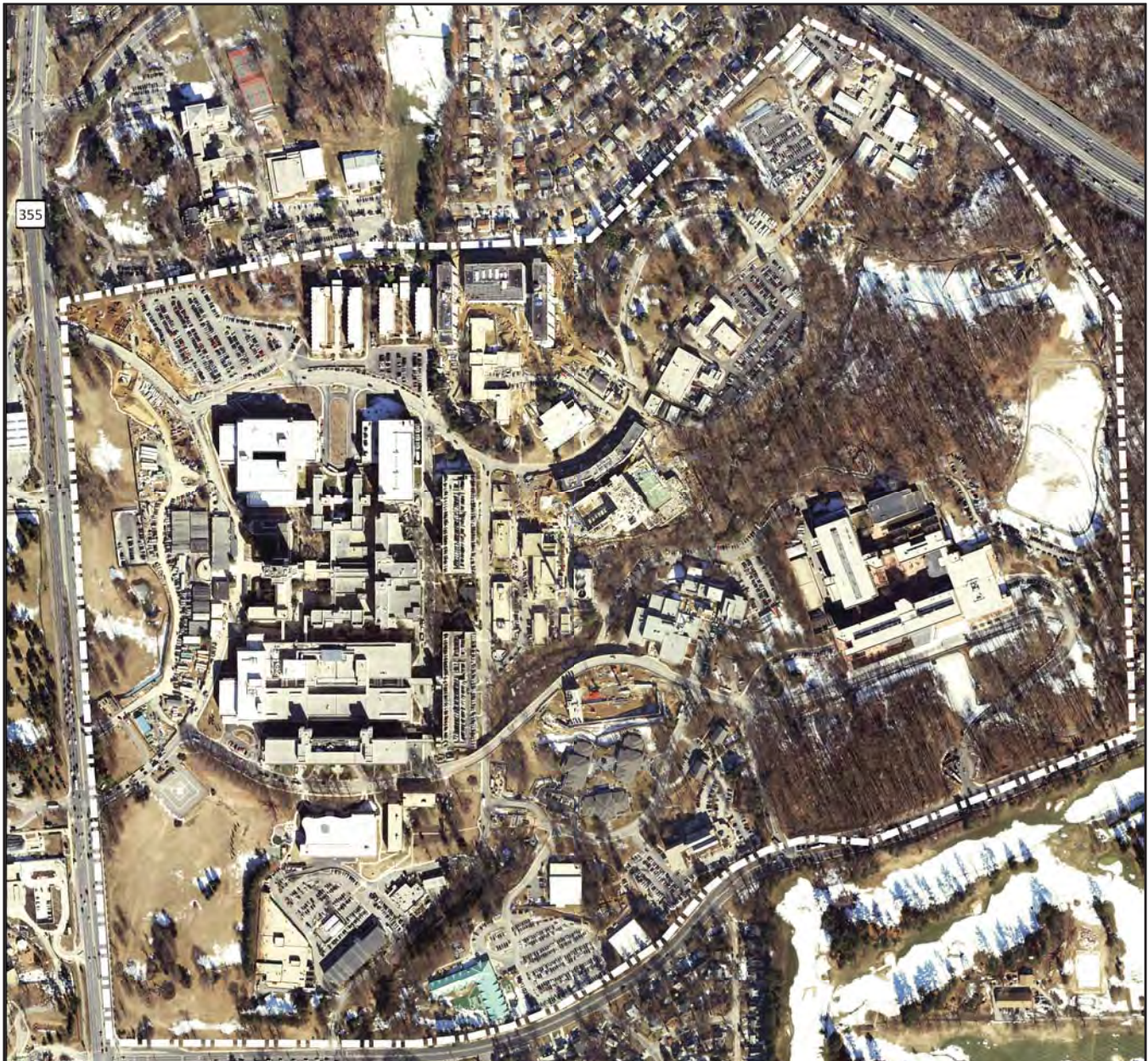
FIGURE 4-1 SITE OVERVIEW AERIAL
