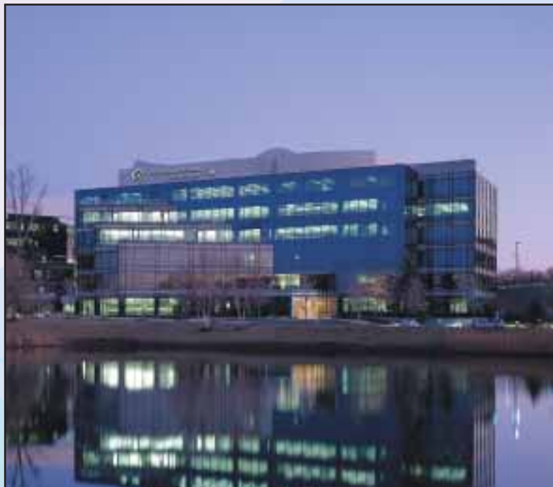
CFC — the Herndon, Va., headquarters of which is seen here — is the primary private market lender to rural electric systems serving more than 32 million consumers. Photo courtesy CFC
