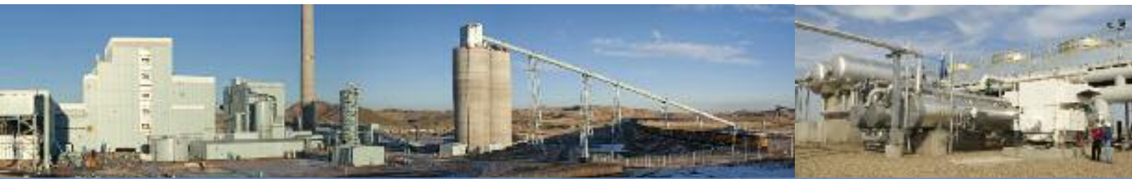
Basin Electric's Dry Fork Station near Gillette, Wyo., is the co-op's newest power plant.
