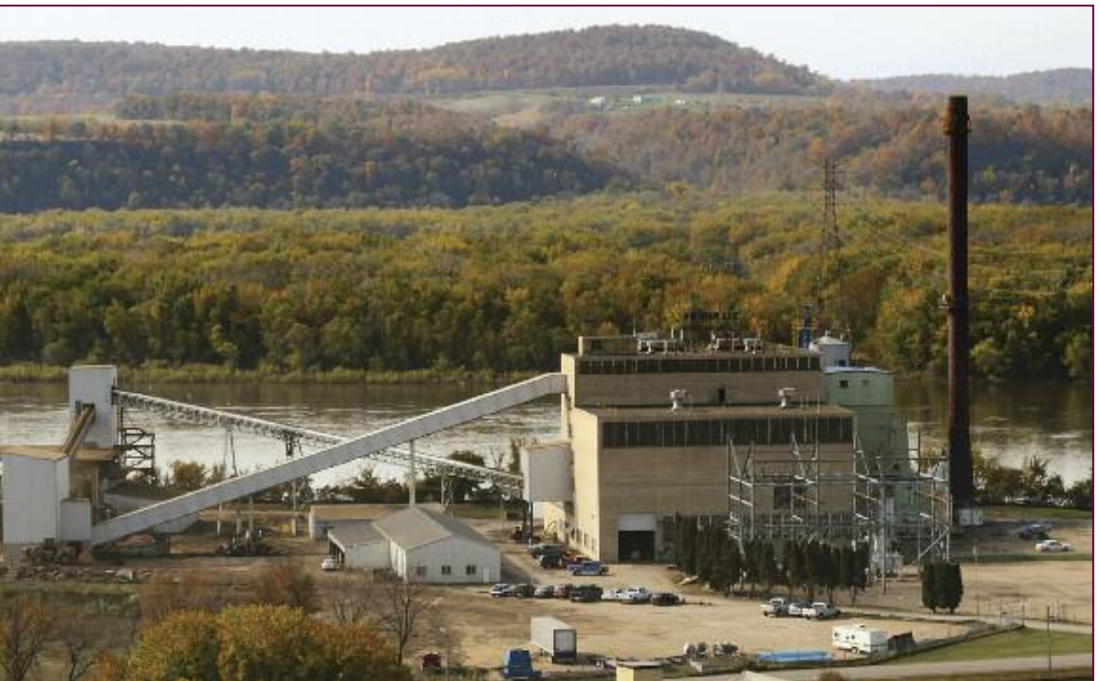
This Dairyland Power Cooperative (DPC) plant, which formerly burned coal, now runs on 1,000 tons of biomass daily. Photo courtesy DPC
