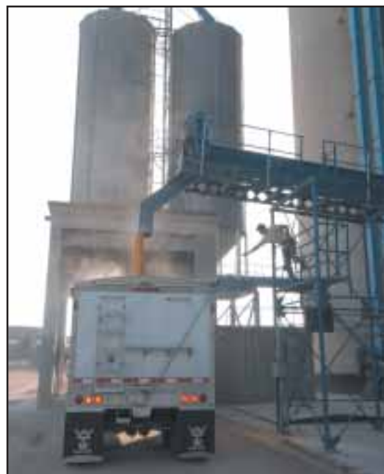
All 27 of CHS’ “regionalized” local co-ops retain daily operational authority, but the CHS board decides the percentage of cash patronage refunds and the level of equity redemption. Above, grain loading at the Corson Co-op in southeastern South Dakota. Photo courtesy CHS.
