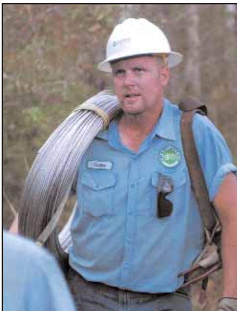
Employees from Poplar Bluff, Missouri's Ozark Border Electric Cooperative and other out-of-state co-ops had to adapt to working in Florida's high humidity, soft sandy soil and marshes.
