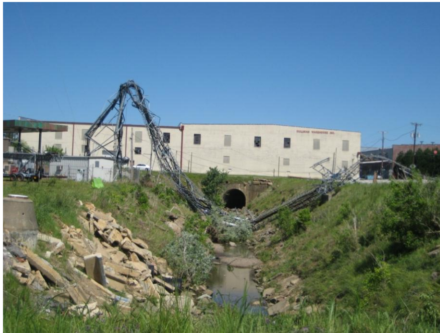
Figure 7: Destroyed NWR transmitter tower at Cullman, AL (courtesy of WFO Huntsville, AL)
