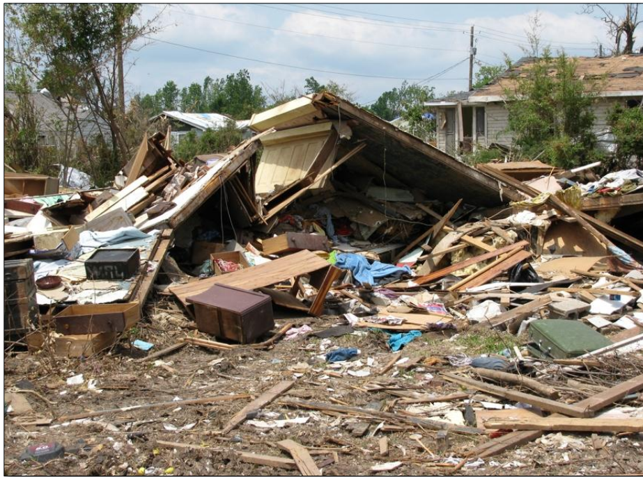
Figure 16: A destroyed wood frame house in Concord, AL (courtesy of Gary Woodall, MIC, NWS Phoenix, AZ)
