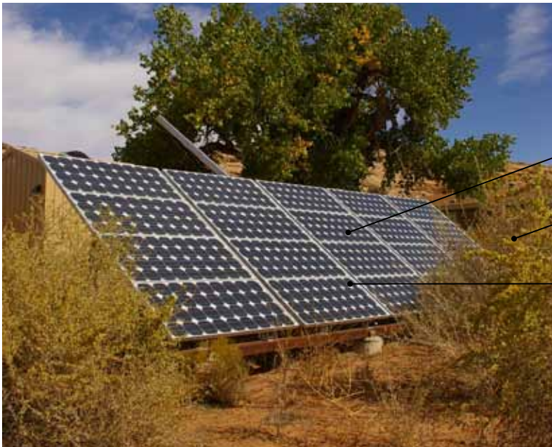
Sand Island Recreation Area, Utah
