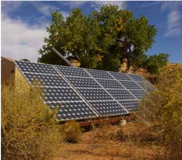
Sand Island Recreation Area, Utah
