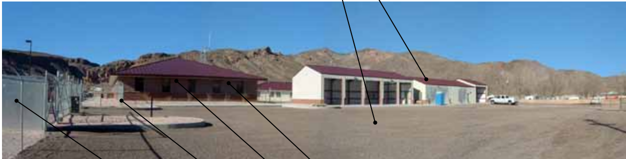
Caliente Maintenance Wareyard, Nevada
