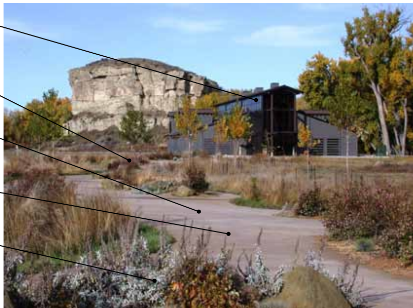
Pompeys Pillar National Monument Interpretive Center, Montana
