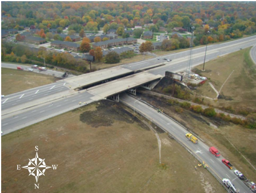
Figure 8. Aerial view of the connection ramp and Interstate 465 overpasses. (Source: Indiana State Police.)
