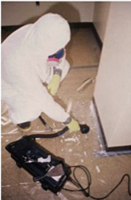
FIGURE 14.8 Vacuuming the floor containment.
