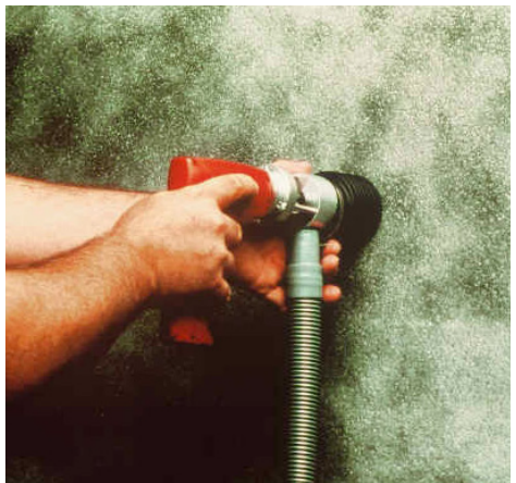
FIGURE 12.19 Needle Gun with HEPA Exhaust Ventilation.
