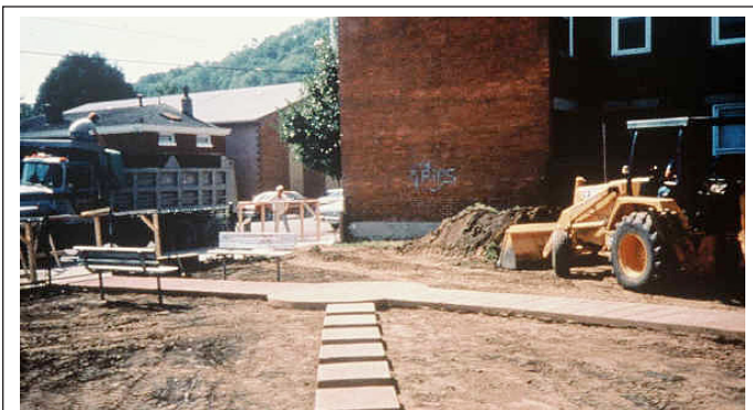
FIGURE 12.22 Replacing resident pathway after soil removal.
