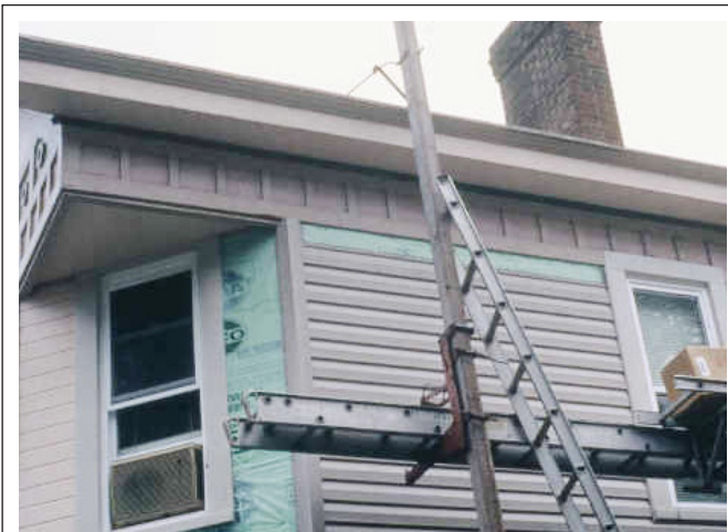
FIGURE 12.6 Installation of replacement siding.
