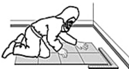
FIGURE 12.10 Install underlayment and new flooring as a suitable LBP enclosure method. The personal protective equipment is for a high-dust project.
