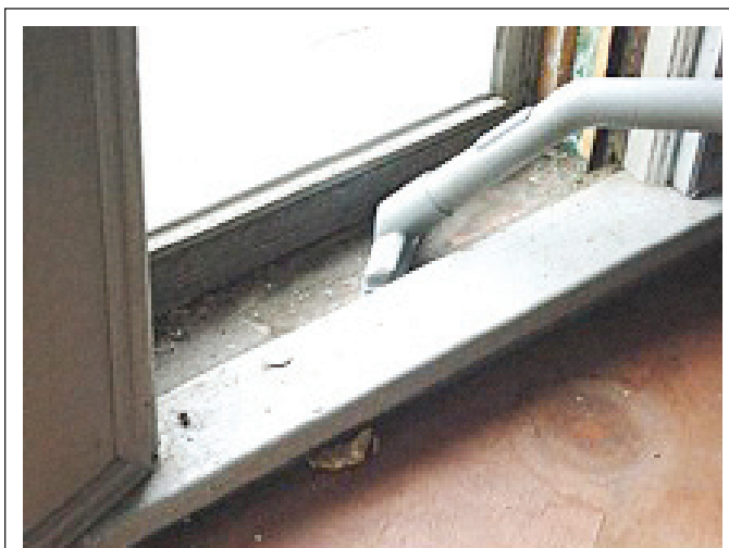
FIGURE 11.5 Prepare the worksite and pre-clean the window.
