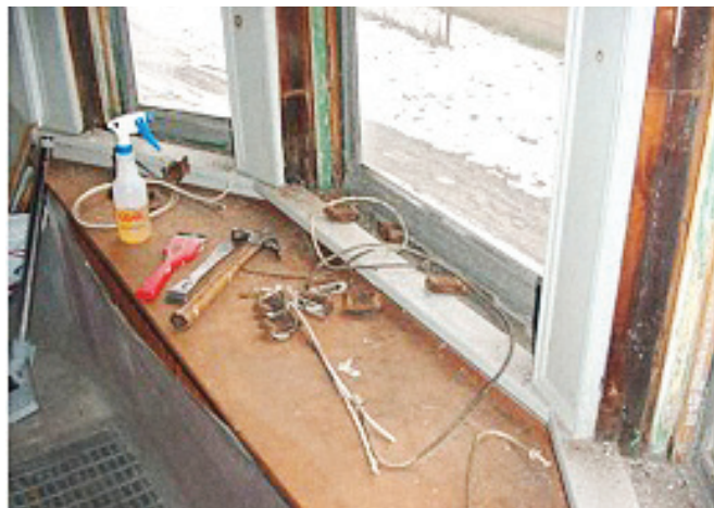
FIGURE 11.9 Window after removal of sash weights.
