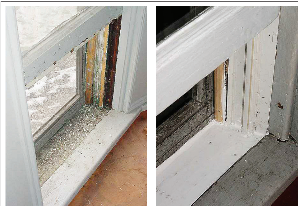
FIGURE 11.3 Window before and after friction treatment.
