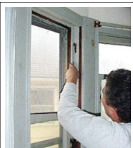
FIGURE 11.6 Remove parting Bead.
