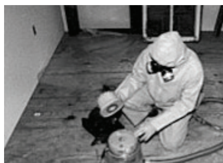
f) Remove & Replace HEPA Filter Assembly.
