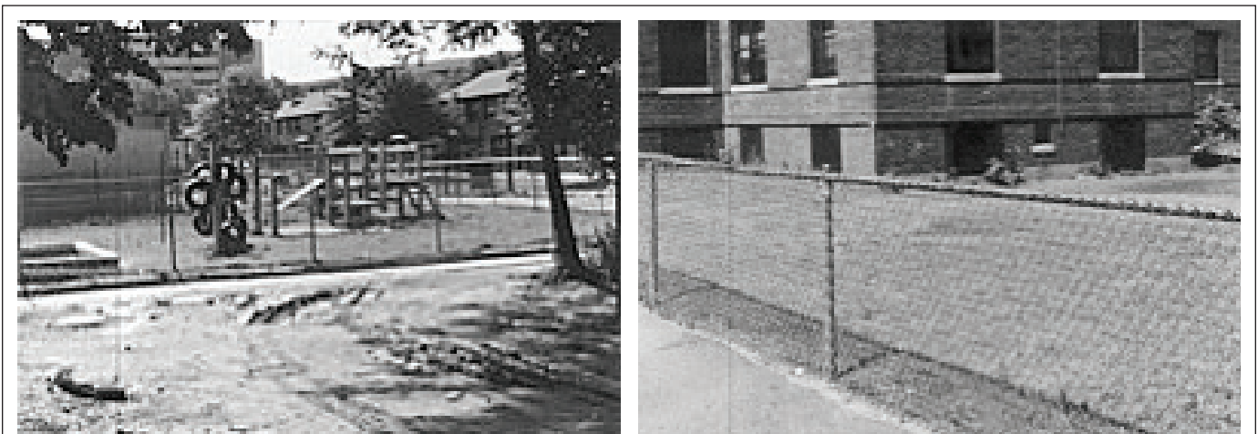
FIGURE 11.28 Using Fencing as an Interim Control. a) For Bare Soil. b) For other soil.
