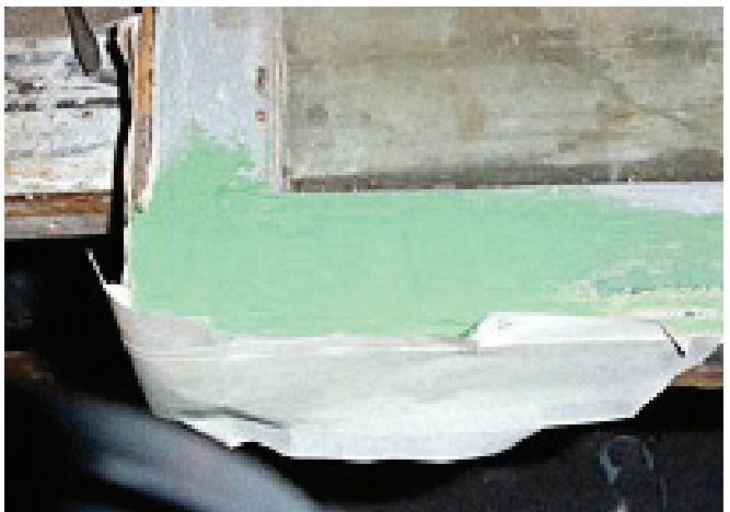
FIGURE 11.10 Rebuild damaged sash with filler or putty.
