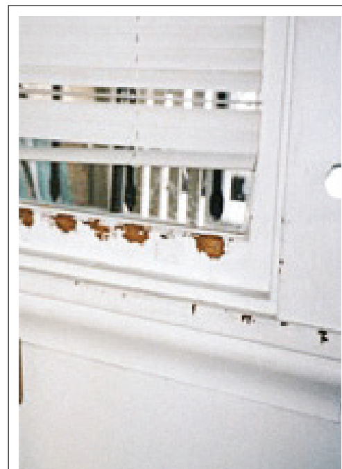
FIGURE 5.8 Chewable surface: teeth marks on window sill.
