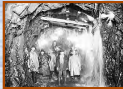
Difficult working conditions
