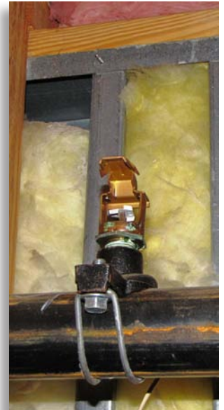
This attic special sprinkler is designed to be installed near the ridge of a peaked attic and can project water up to 40 ft (12.1 m).
