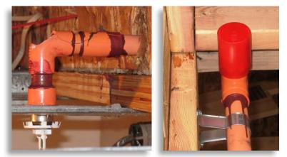
These pictures reveal careless work on behalf of the sprinkler fitter joining nonmetallic pipe and fittings. Photos courtesy of Keith Heckler, Rockville Fire Department, MD.
