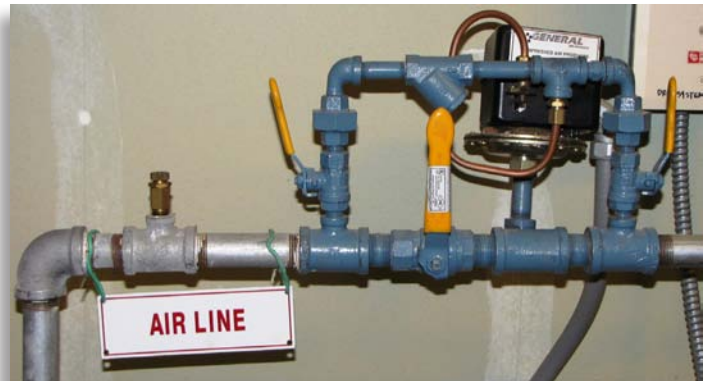
This listed assembly is designed to maintain a stable air pressure on the system side of a dry-pipe valve to prevent accidental trips.
