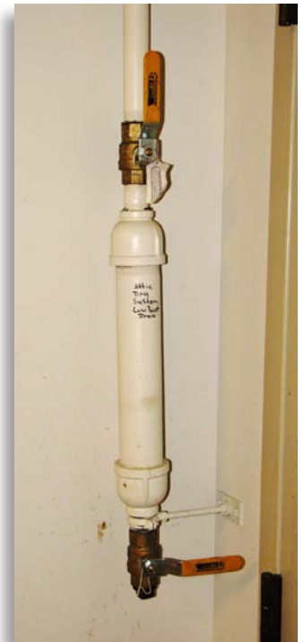
The low point drain assembly also may be called a “drum drip.”
