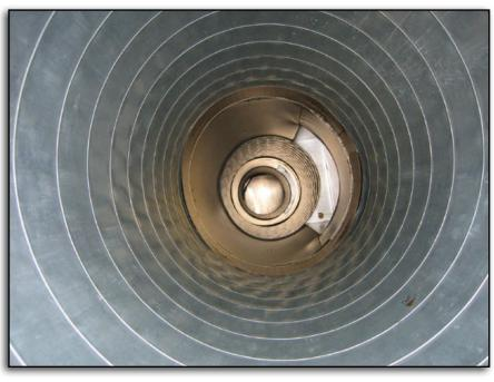
Photo courtesy Keith Heckler, P.E., Rockville Fire Department, Maryland. This laundry chute must be sprinklered to prevent vertical fire spread.
