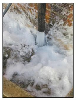
If not controlled, the discharge from the main drain can create significant damage.
