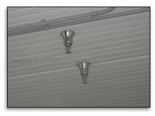
These sprinklers should have a baffle between them. Photo courtesy Minnesota State Fire Marshal's Office.
