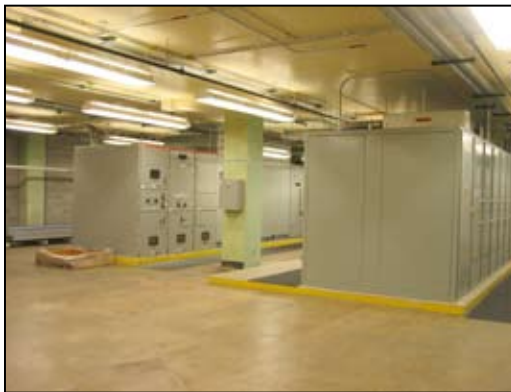
Photo courtesy of Clyde Pfisterer, Indianapolis, IN.
