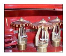
The sprinklers must correspond to the types and temperature ratings of the sprinklers in the property, so if there are standard spray uprights, quick response pendants and Early Suppression Fast Response (ESFR) like those pictured, a representative inventory of each must be provided.
