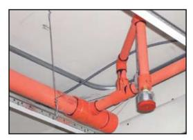
PEX is listed only for multipurpose piping systems (potable and fire protection) in one- and two-family dwelling and manufactured homes. The pipe must be installed with a thermal barrier between the room and the PEX.
