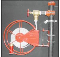
If a sprinkler system has no inside hose stations connected to it, the applied value is "0". If the sprinkler system has one inside hose station, the designer must add 50 gallons per minute to the water supply requirements for the sprinkler system.
