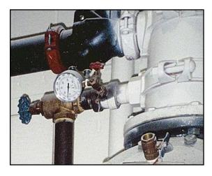
Because of potential turbulence, attaching the gauge to the main drain outlet as shown will result in inaccurate pressure readings during the main drain test. Having the gauge installed here will produce pressure readings that suggest an excessive pressure drop.
