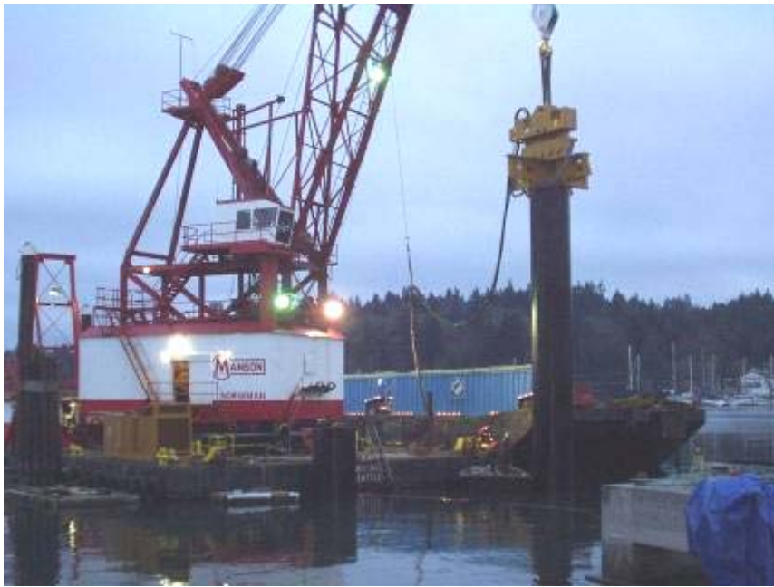
Figure 1-4. Vibratory Installation of Drilled Shaft Casing.
