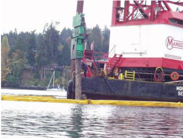
Figure 1-8. Vibratory Hammer Removing a Timber Pile.
