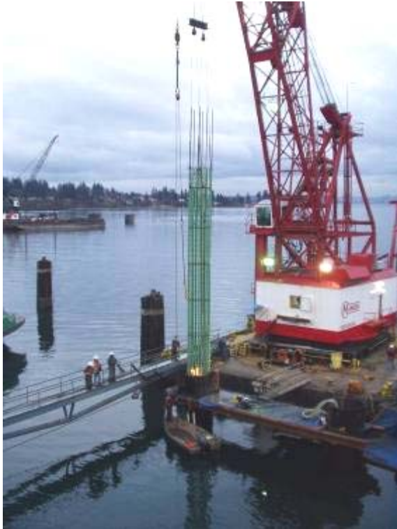
Figure 1-6. Rebar Reinforcement of Drilled Shaft.
