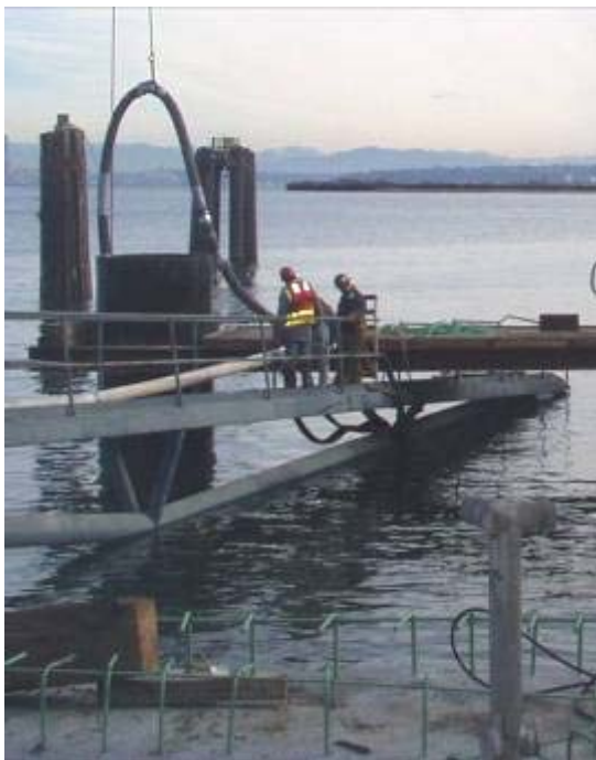
Figure 1-7. Vacuuming of Slurry from Drilled Shaft.
