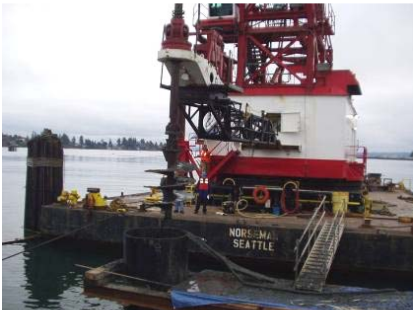
Figure 1-5. Auger Excavation of Drilled Shaft.
