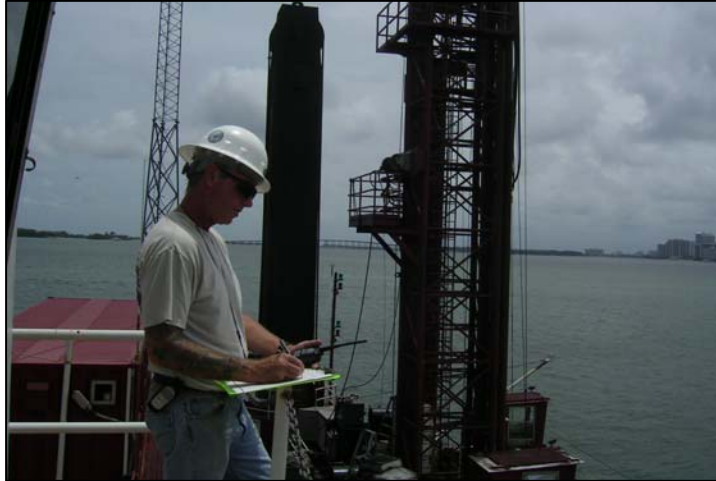
Figure 24: Observer on the drill barge.
