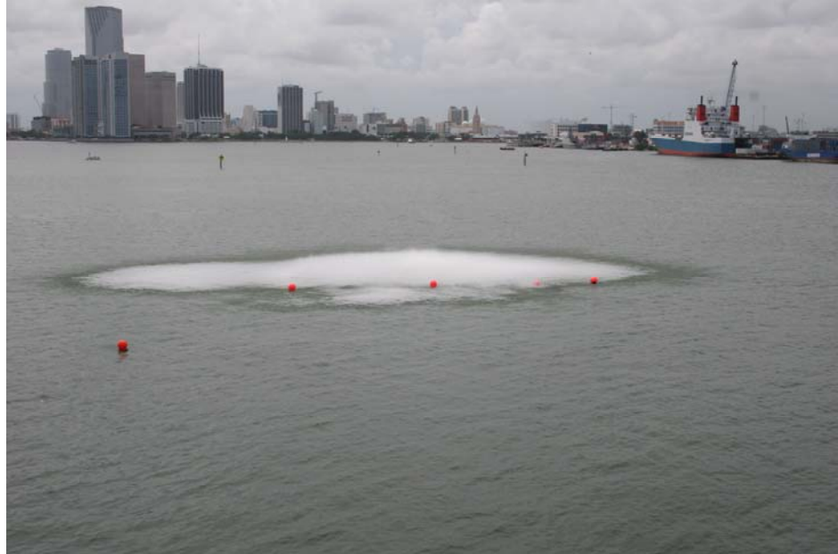
Figure 7 - Confined blast of 3,000 pounds
