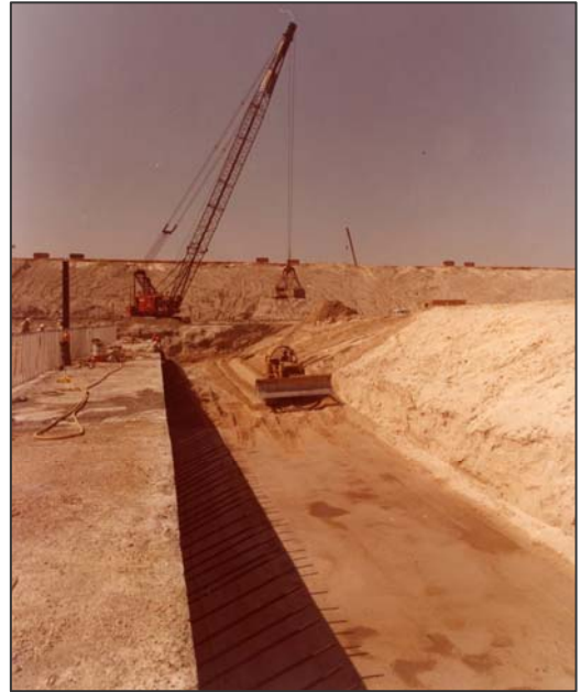
Figure 4: Concrete sill under construction – note extensive rebar.
