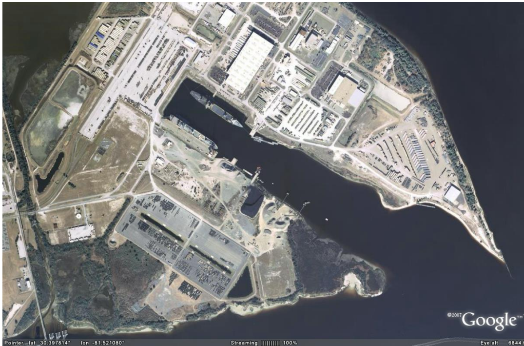
Figure 2: MSCF-BI facility overview
