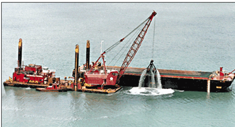
Figure 8: Mechanical dredging; clamshell dredge with scow. (Photo: Great Lakes Dredge & Dock Co.)
