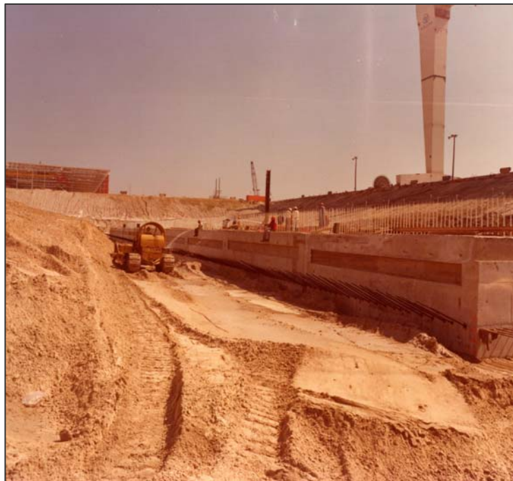
Figure 5: View from top of concrete sill; note extensive rebar.
