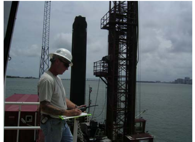
Figure 10: Observer on the drill barge
