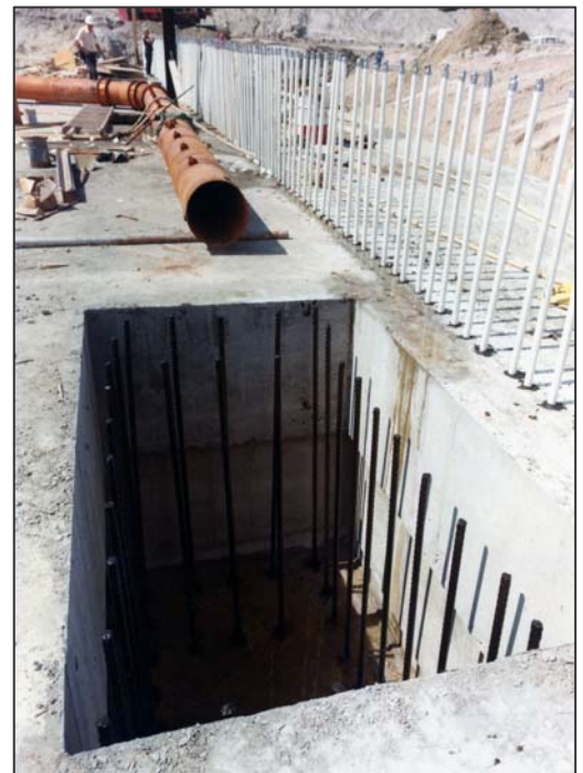
Figure 6: Rebar reinforcement of – concrete sill.
