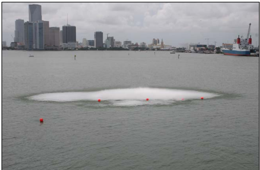
Figure 22: Confined blast of 3,000 pounds of explosives.
