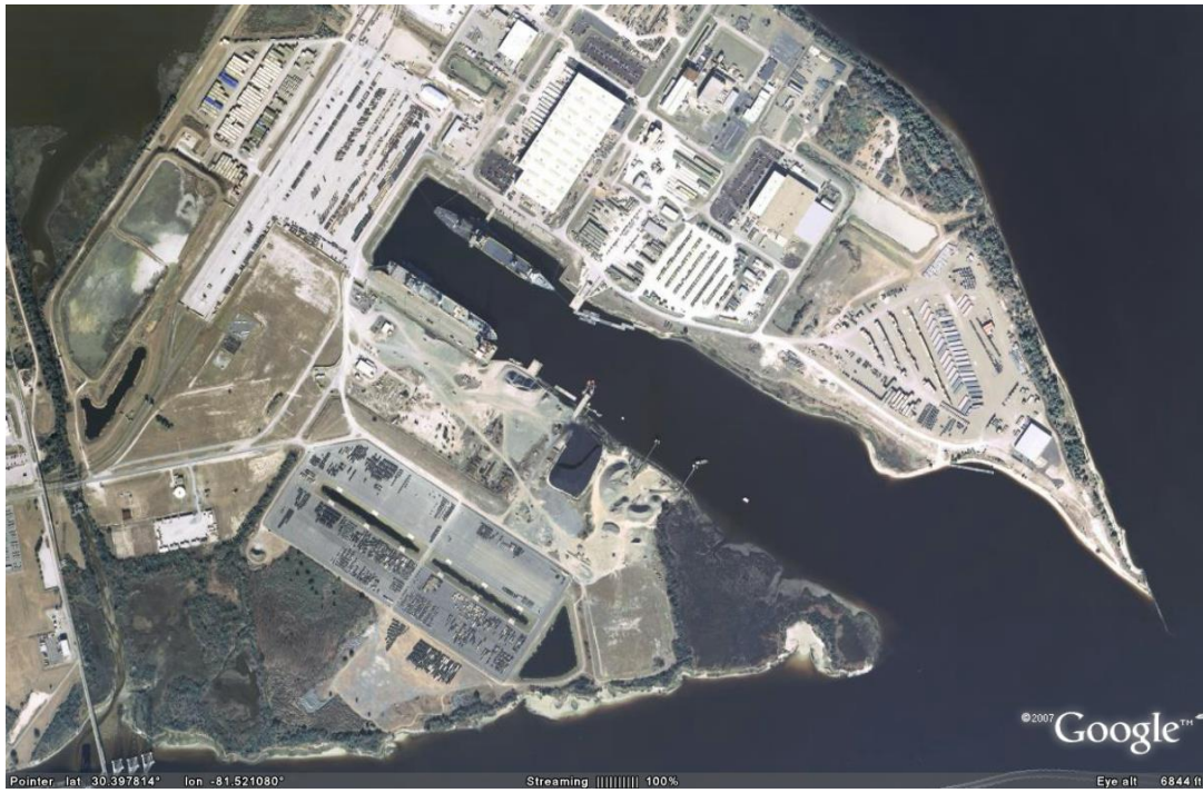
Figure 2: MSCF-BI facility overview
