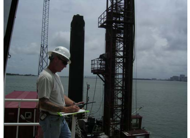
Figure 10: Observer on the drill barge
