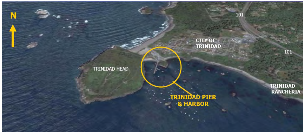
Figure 1-1. Oblique aerial photograph of project area
