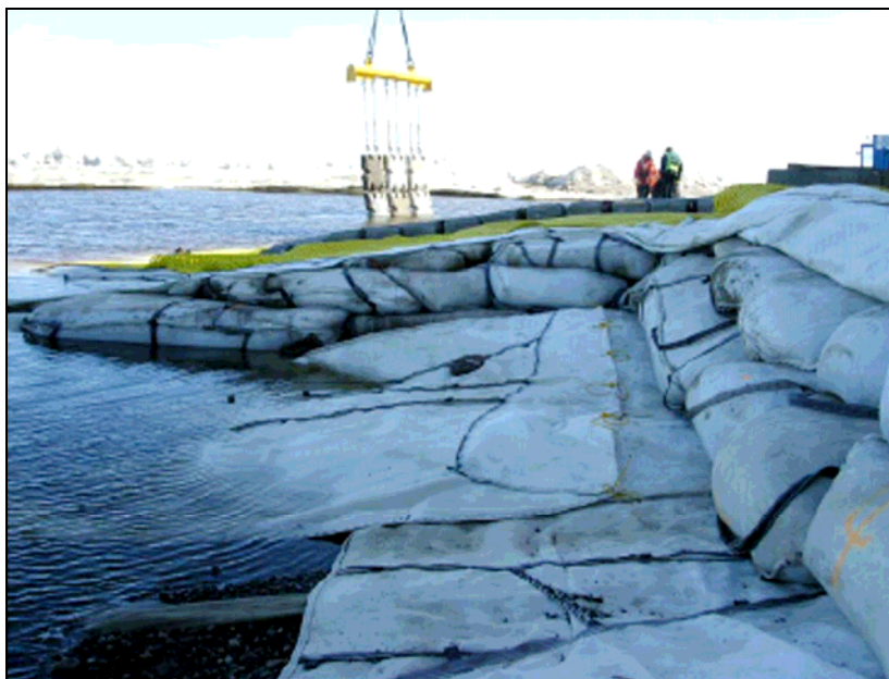
FIGURE 1.7. Gravel bags used to build up elevation of Northwest corner.
