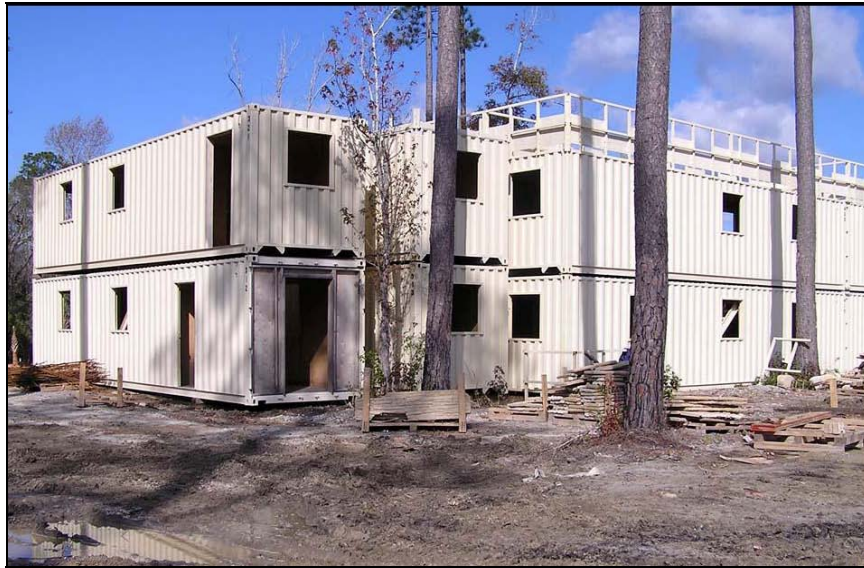
Example of Prefabricated Metal Containers to be erected at Airfield Seizure Facility on MCOLF Atlantic
