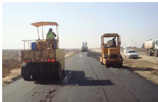
Workmen pave the Al Amarah-Al Maymunah Carriageway. (USACE photo)
