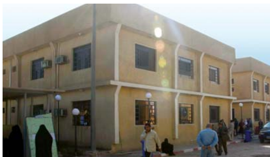
U.S.-funded upgrades to the Sadr City Courthouse include shatterproof and bulletproof windows, as well as new safety lighting. (USACE photo)
