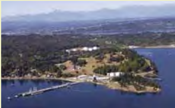
FLC Puget Sound Fuel Department is a 234-acre site in eastern Kitsap County, Washington. It contains approximately two miles of Puget Sound shoreline and a 26-acre lagoon.
