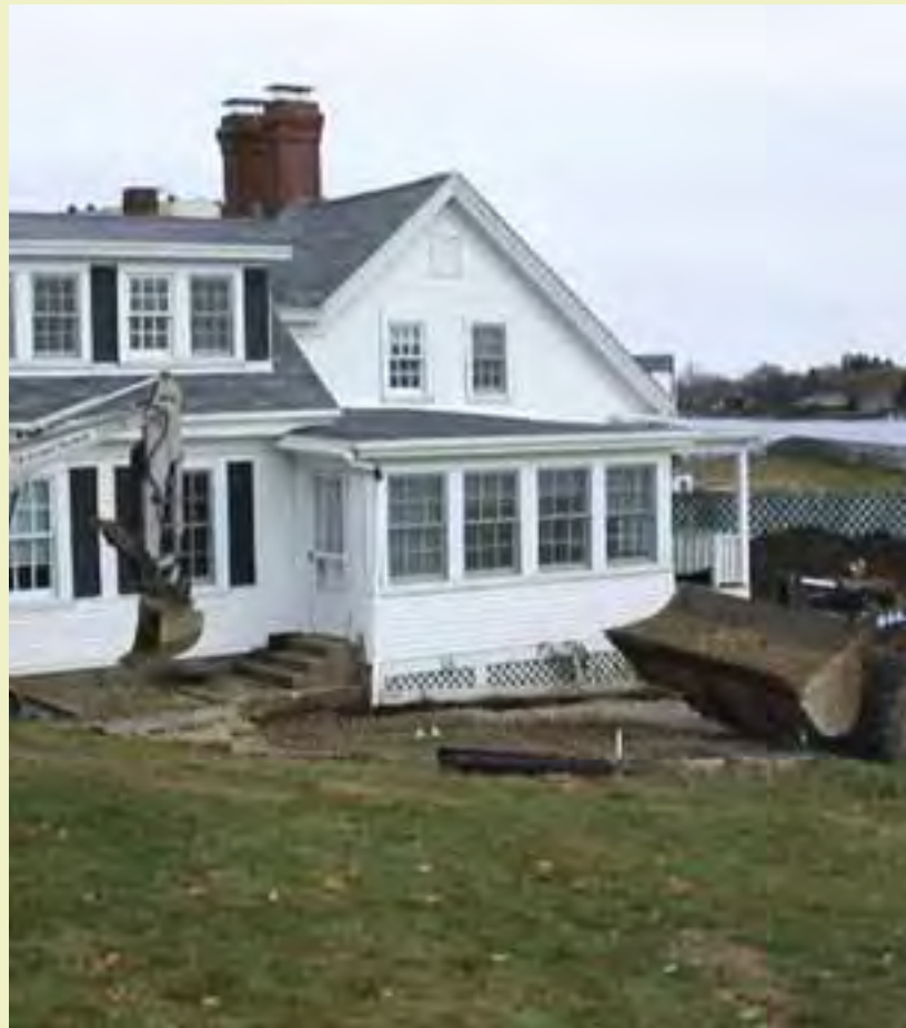
After soil sampling activities were completed at PNSY, each area was backfilled with gravel, lined with geotextile fabric, and top dressed with loam and seed. Final backfilling, landscaping, and fence replacement were completed during fall 2010 and spring 2011.
