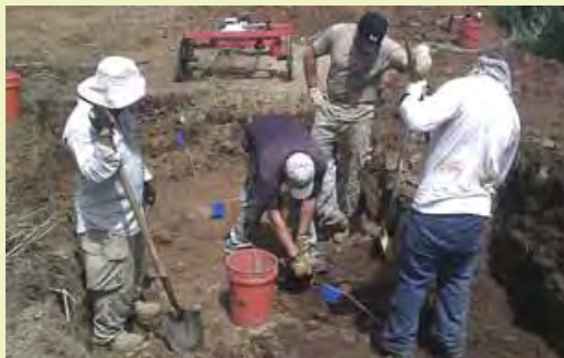
In an effort to locate subsurface MEC, a geophysical instrument (in background) is used to identify the location of metallic anomalies that may be indicative of munitions. Technicians then dig out the anomalies to identify and remove (or detonate) the munitions.
