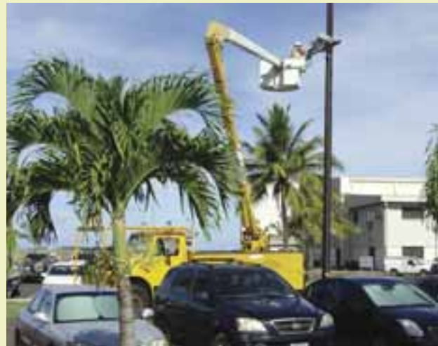
In an effort to minimize fallout of protected nocturnal migratory seabirds, lamps at Barking Sands beach are being changed to test the efficacy of Light Emitting Diode (LED) lights. These changes are expected to aid fledgling migration and save energy.
