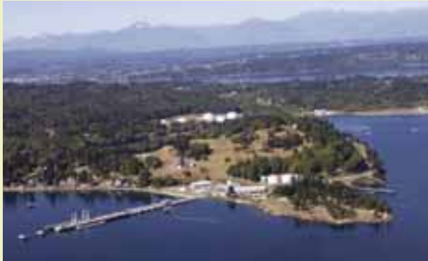
FLC Puget Sound Fuel Department is a 234-acre site in eastern Kitsap County, Washington. It contains approximately two miles of Puget Sound shoreline and a 26-acre lagoon.
