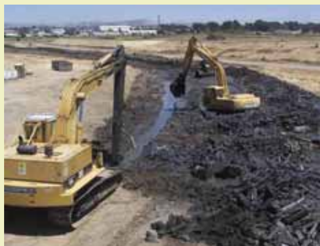
A 7,300-foot long slurry wall surrounding the Investigation Area H1 containment area prevents contamination from migrating into the surrounding groundwater.
