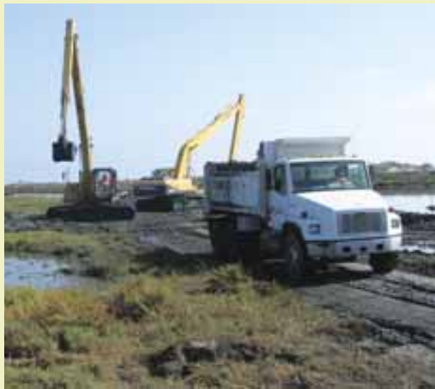
Slag and ash residue is removed from a NBVC Point Mugu lagoon. It took six weeks to remove the ash and slag residue, which totaled almost 2,000 cubic yards.
