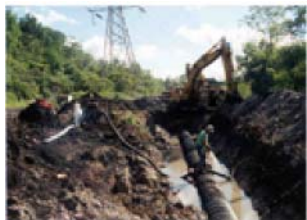
Dewatering pipeline trench
