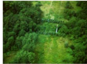
Aerial view of completed pipeline right of way
