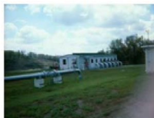
Compressor station building
