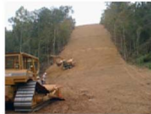
Final grading of pipeline right of way
